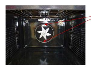
REMOVE THE 2 ELEMENT SECURING SCREWS AND PULL ELEMENT FORWARD INTO THE CAVITY
